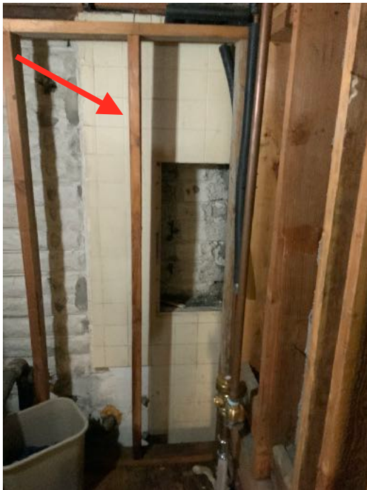
Utility/Storage - Remnant Wall Tile With High Lead Content
