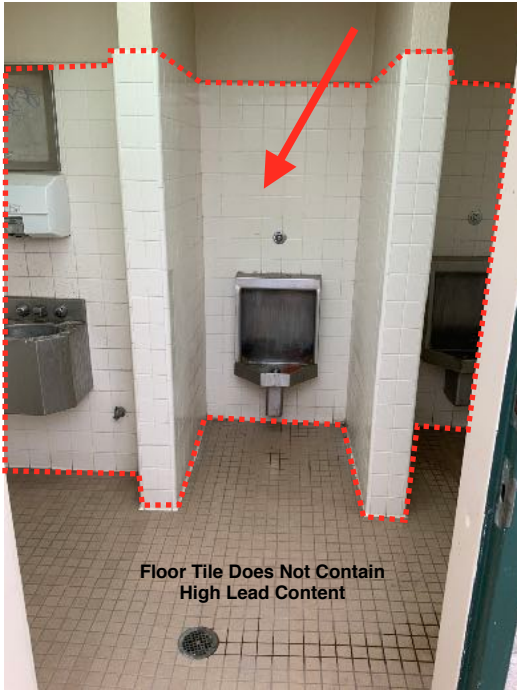
Men's Restroom - Wall Tile With High Lead Content
